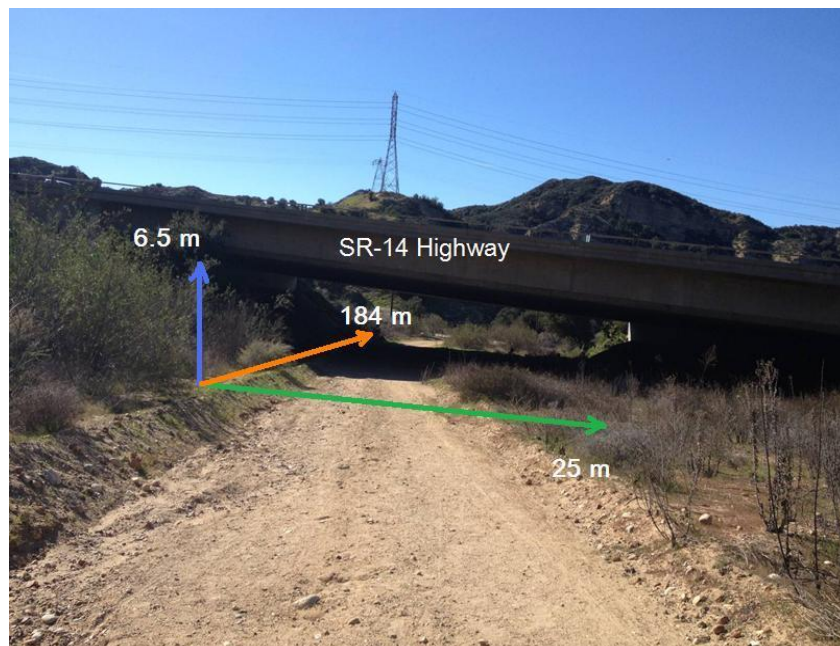
Figure 2: Photo and dimensions of the Los Piñetos underpass and SR-14 facing west.
