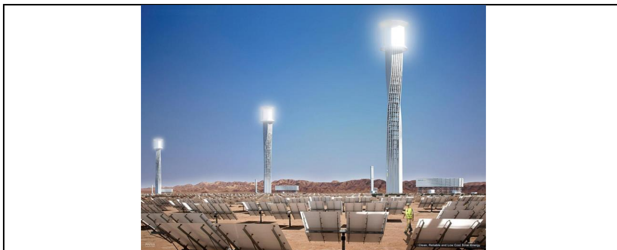
Figure 3.3. This is the Ivanpah solar thermal power plant in the Mojave Desert. It produces 377 MW of energy using a power tower design. 12
