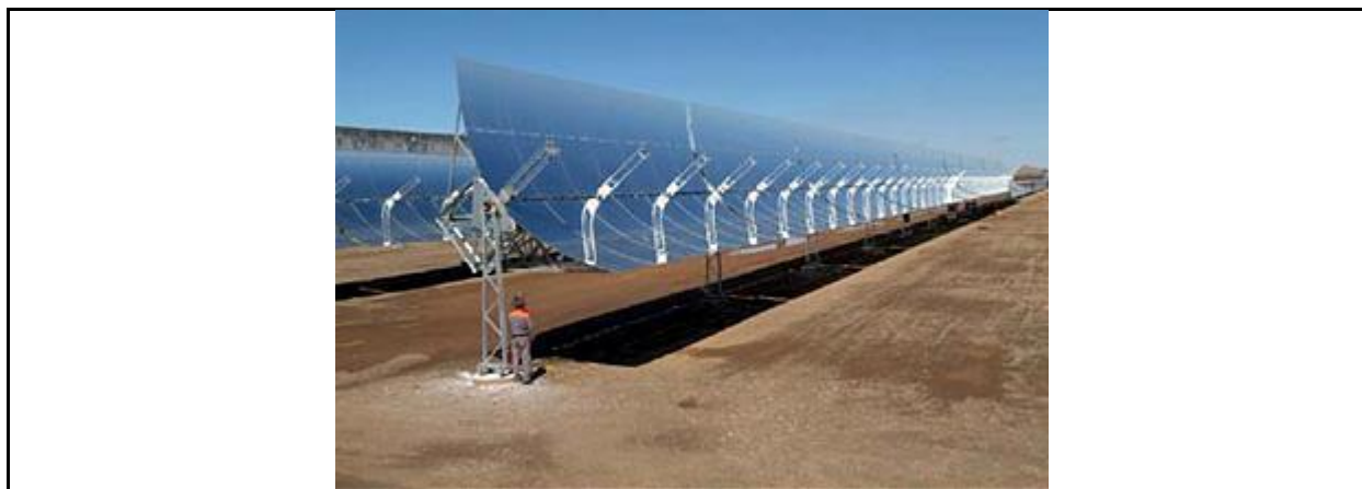
Figure 3.4. This is the Genesis Solar Power Project located in Riverside County. It produces 250 MW of electricity using a parabolic trough design. 15
