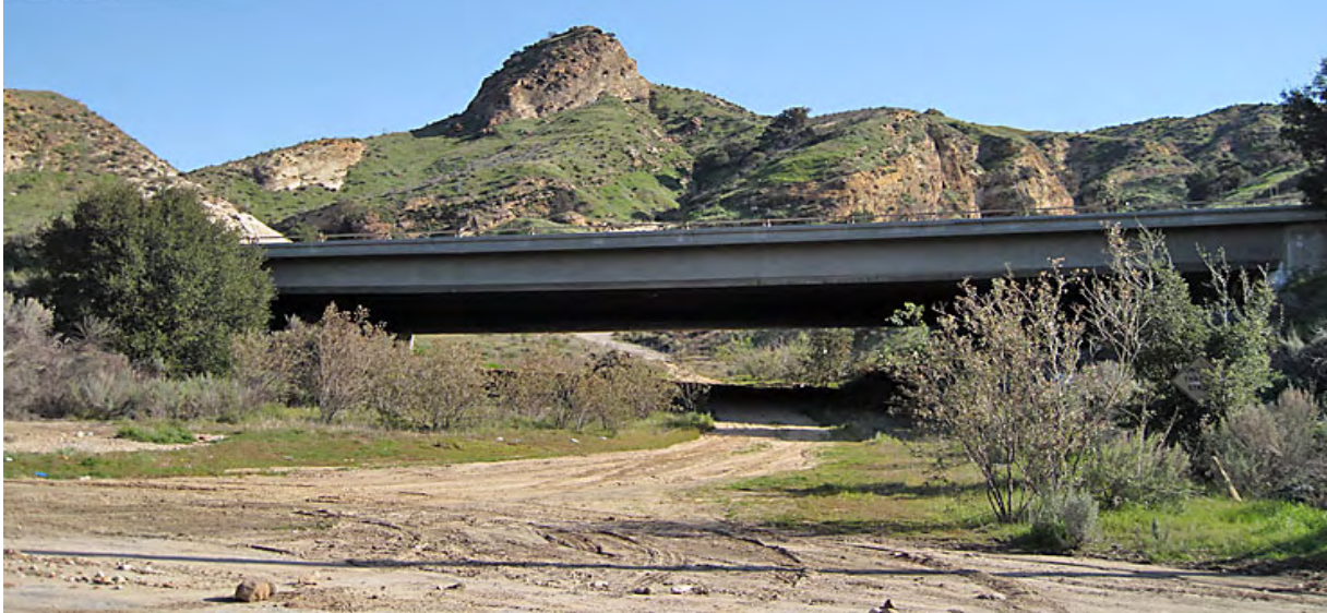
Figure 2. Los Piñetos Road underpass under SR 14, 1.2 miles east of Interstate 5 in Santa Clarita, California.
