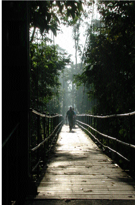
Bridge at La Selva
