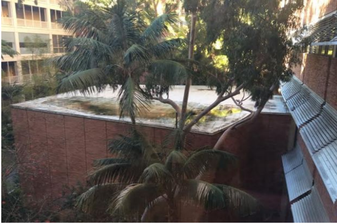
Figure 4: Boelter Hall Interior Courtyard. The cistern will be placed around the protruding lecture hall.
