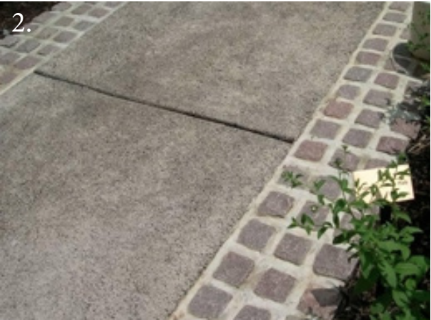
1. Rain Garden in Pacoima Wash Nature Park 2. Pervious concrete walkway bordered by paving stones 3. Storm Drain Screen Cover
