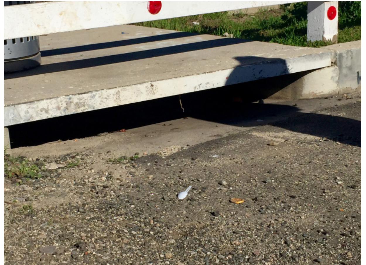
Catch basin without a catch basin screen
