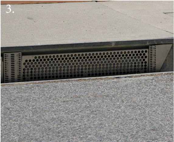
1. Rain Garden in Pacoima Wash Nature Park 2. Pervious concrete walkway bordered by paving stones 3. Storm Drain Screen Cover
