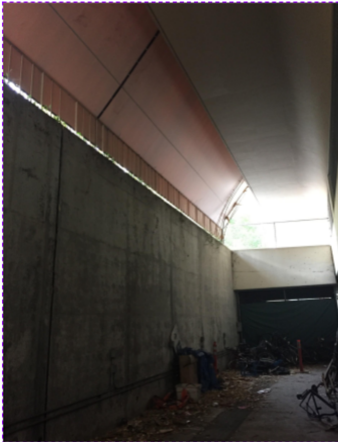
Figure 2: Photograph of the Parking Structure 9 site location from ground level.
