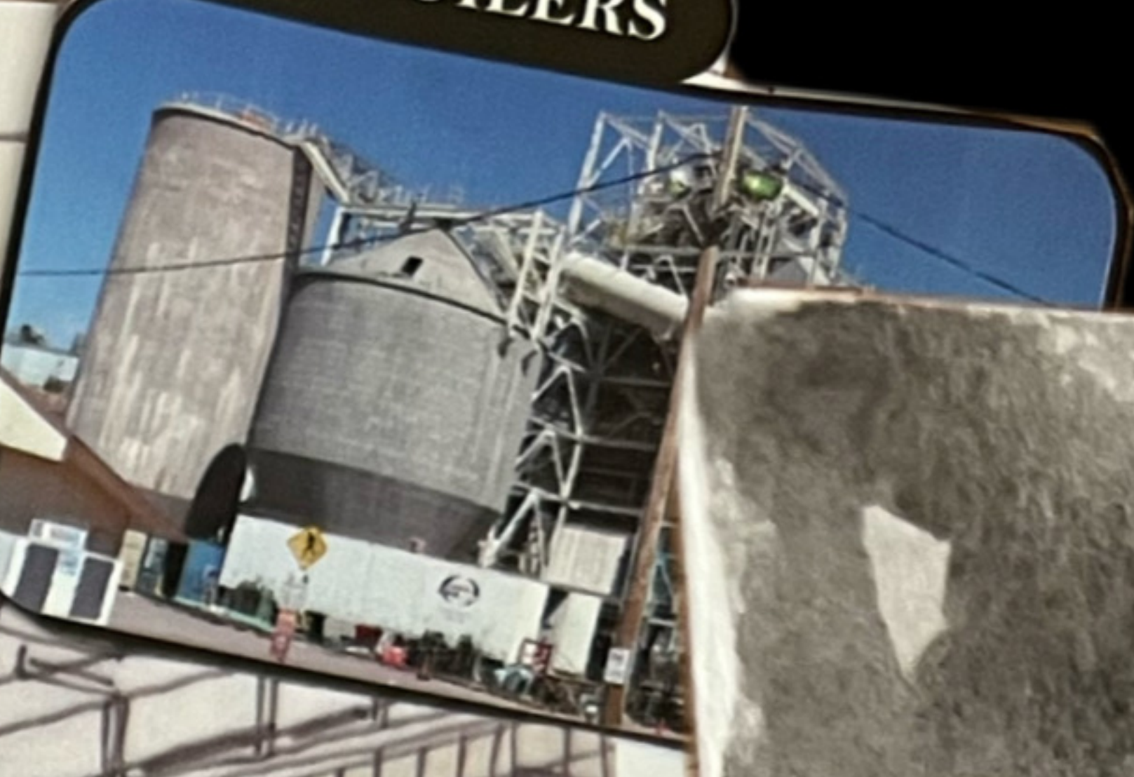
C BIOMASS BOILERS
