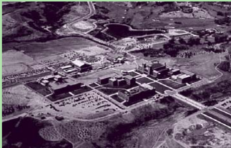
This 1932 aerial photograph shows the eastern arroyo in the foreground, with western arroyo and Faculty Ridge in the upper left. The eastern arroyo was filled in 1947, while the western arroyo (Sunset Canyon) remained native habitat until the 1980s.
