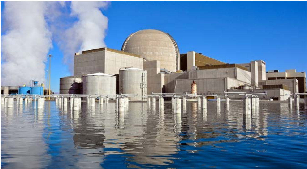
The Palo Verde Generating Station near Tonopah, Arizona. (photo credit: photo from LinkedIn).
