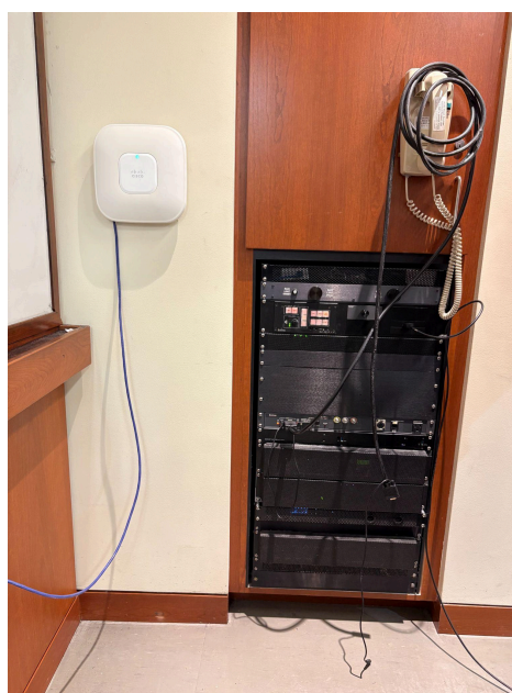
Figure 2. Wifi Router and Embedded AV Machine with Exposed Wiring in PAB 2434
