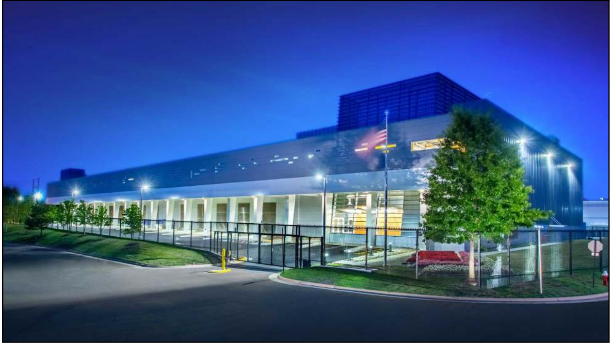
Data Center Campus in Ashburn, Virginia*
