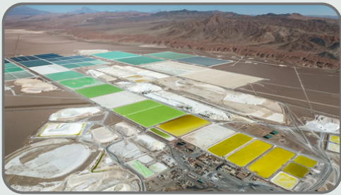
Lithium evaporation ponds in the Salar de Atacama
