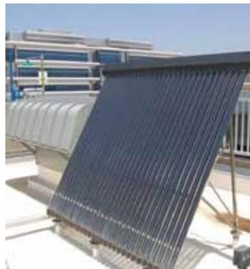
ELC's roof also has many sustainable features. The building's green roof is irrigated with recycled water, and skylights provide natural light to the second floor. A set of 24 photovoltaic panels – 175 W each – generates electricity to be sent to the grid. A demonstration-size wind turbine also sits on the roof for visitors to see. A solar water heater sitting in the sun preheats the building's hot water, reducing the load on the conventional water heater.
