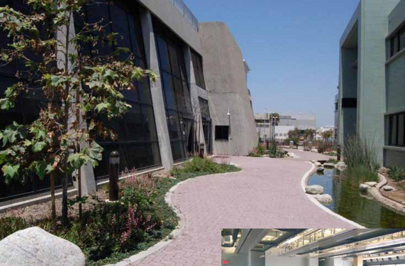
The walkway leading to ELC's entrance is made of permeable pavers to enable percolation of stormwater. The stream along the right is connected to the wetlands, which is supplied by recycled water from the West Basin Municipal Water District, which receives and treats secondary effluent from the Hyperion Treatment Plant. The plants along the path are drought-tolerant native species. Bureau of Engineering
